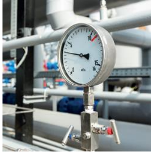
Hydraulic Pressure Testing
